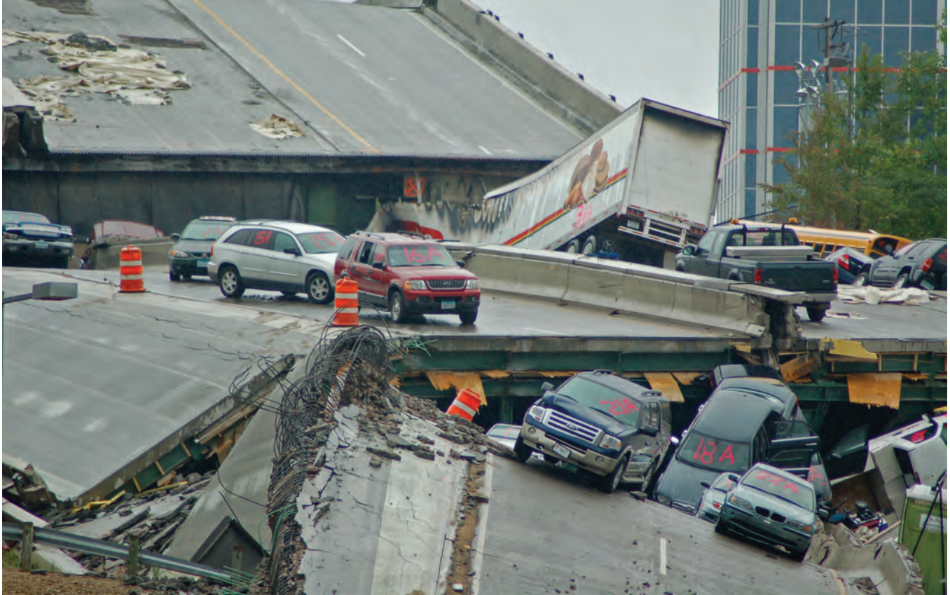
After only 74 years of experience with the element, how well do we really understand plutonium? We still have problems predicting the stability of steel structures under stress, despite our over 2,000 years experience with steel. Here, cars rest on the collapsed portion of the I-35W Mississippi River bridge in Minneapolis, MN, after the bridge's August 1, 2007, collapse. (Photo: Open Source)
